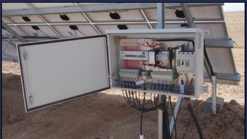
Figure 2 - Junction Box, also known as Combiner Box, which groups wiring from each solar PV module by blocks 2
