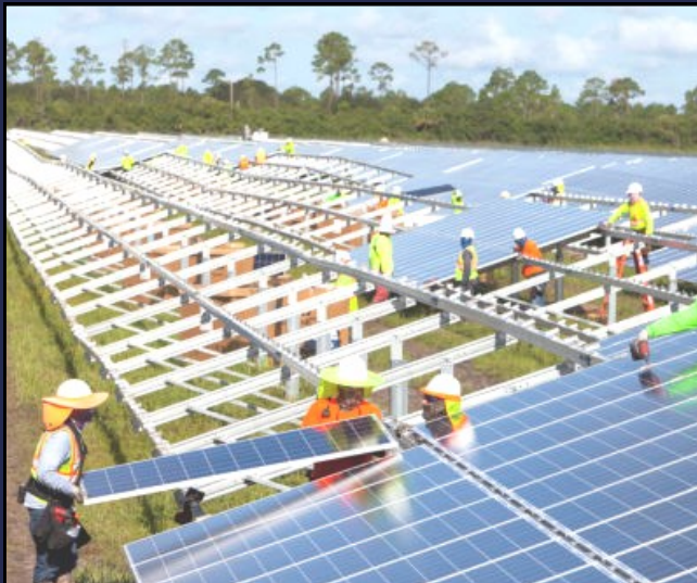
Figure 1 - Workers installing panels at the Babcock Solar Energy project in Punta Gorda, Florida. The project is one of eight new utility-scale solar farms in the state set to be completed by early 2018. FLORIDA POWER & LIGHT 1
